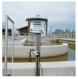
The IQ SensorNet 2020 XT terminal mounted tank side provides continuous process monitoring and control.
