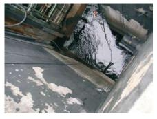
The ultrasonic cleaning capabilities of the ViSolid® and VisoTurb® prevents fouling of the optical sensors. They are installed here in a clearwell to monitor the plants effluent.
